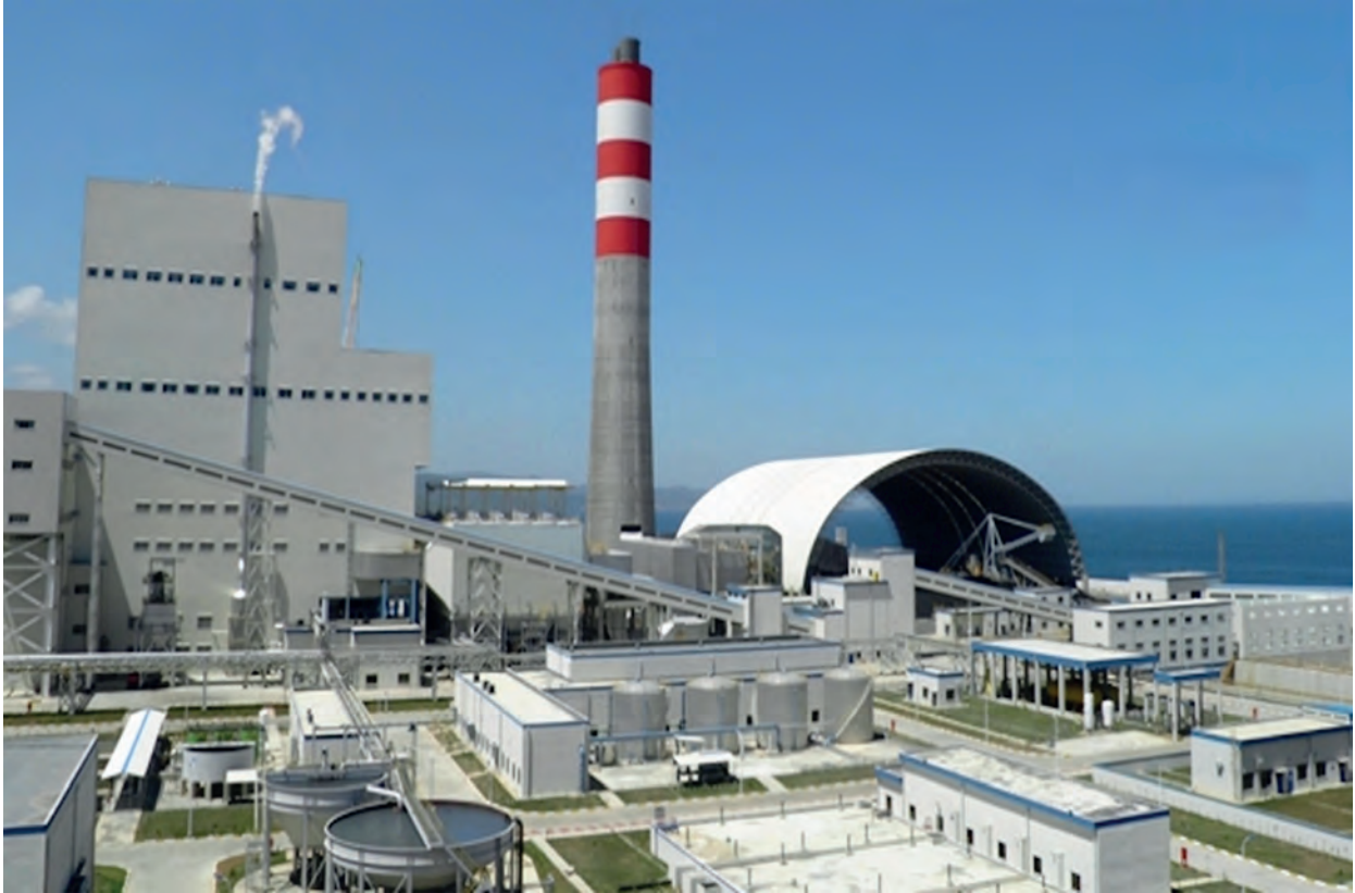
Bekirli Power Plant
