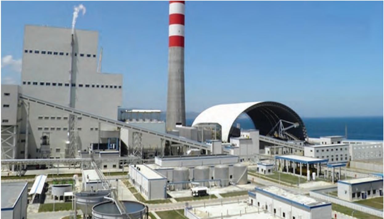
Bekirli Thermal Power Plant
